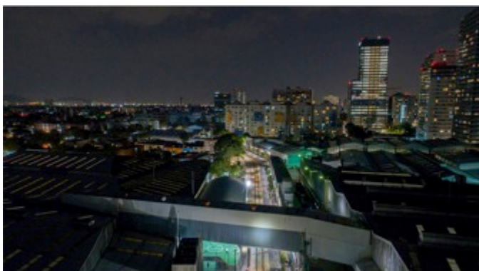
LINEAR PARK CUERNAVACA RAILROAD GAETA-SPRINGALLI ARCHITECTOS from Mexico Photo: Arturo Arrieta, David Cohen
